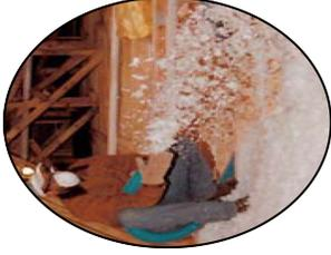
**Ceiling Insulation blown-in R-49 with vapor barrier**
