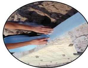
**Cauked perimeter Sill gasket under 2x6 bottom plate**
