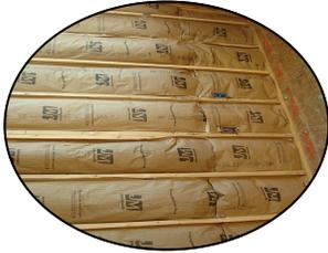
**R-21 batt Insulation with vapor barrier on 2x6 exterior walls 24" on center**
